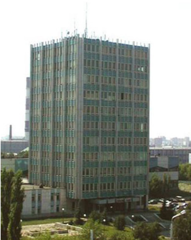
Fig. 3. (Color online) The IMSP building in Ufa used for research on all aspects of superplastic flow and superplastic forming [8].
